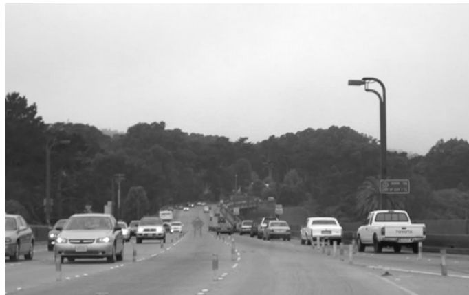
View of Doyle Drive looking west
