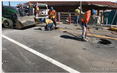
Crews installing drainage
