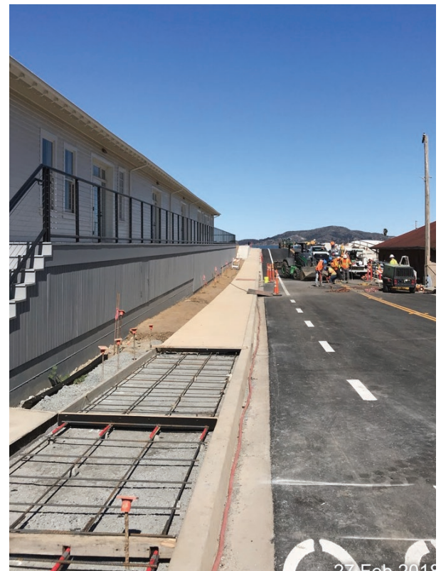
Newly restored Building 201
